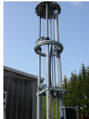
Earth Drilling Rig
